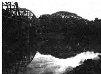
Figure 2. Carmen Bridge Site
