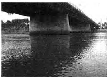
Figure 3. Marcos Bridge (Consolacion) Site
